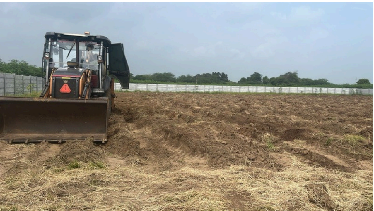
Land Clearing & Levelling
