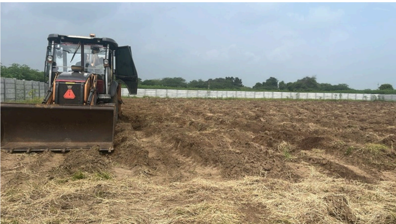
Land Clearing & Levelling
