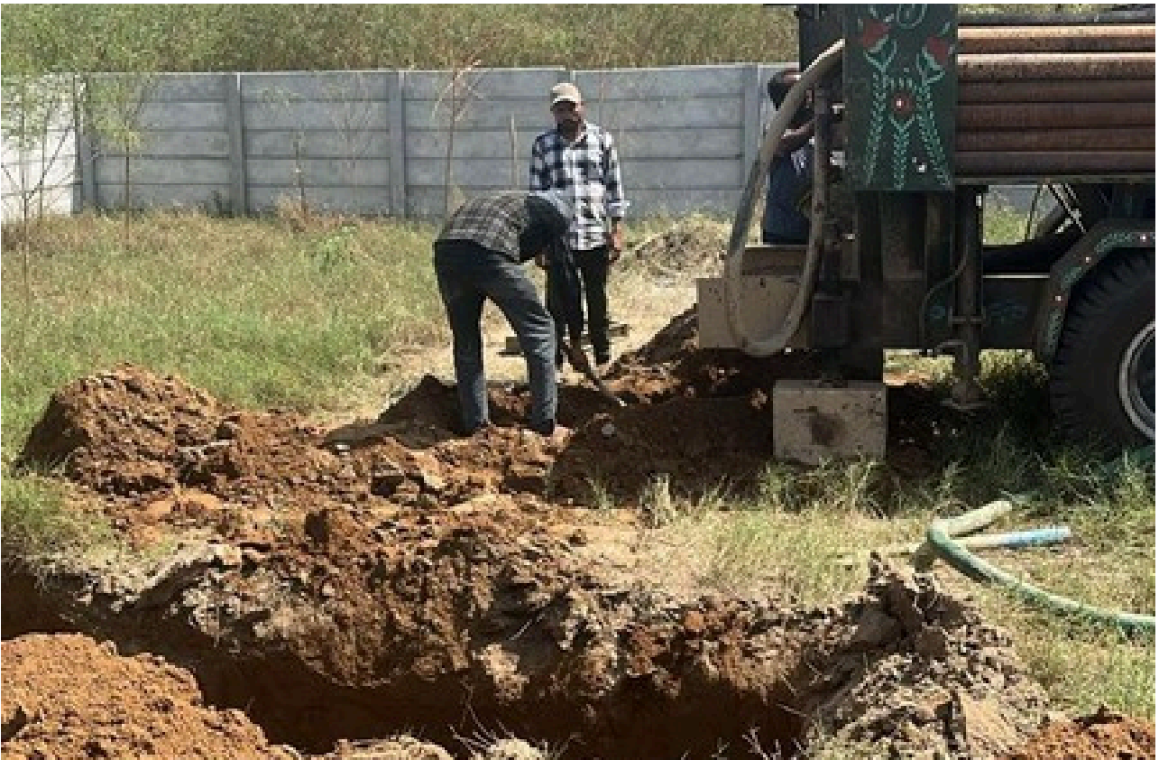
Boring for Submersible Pump (100 Feet)
