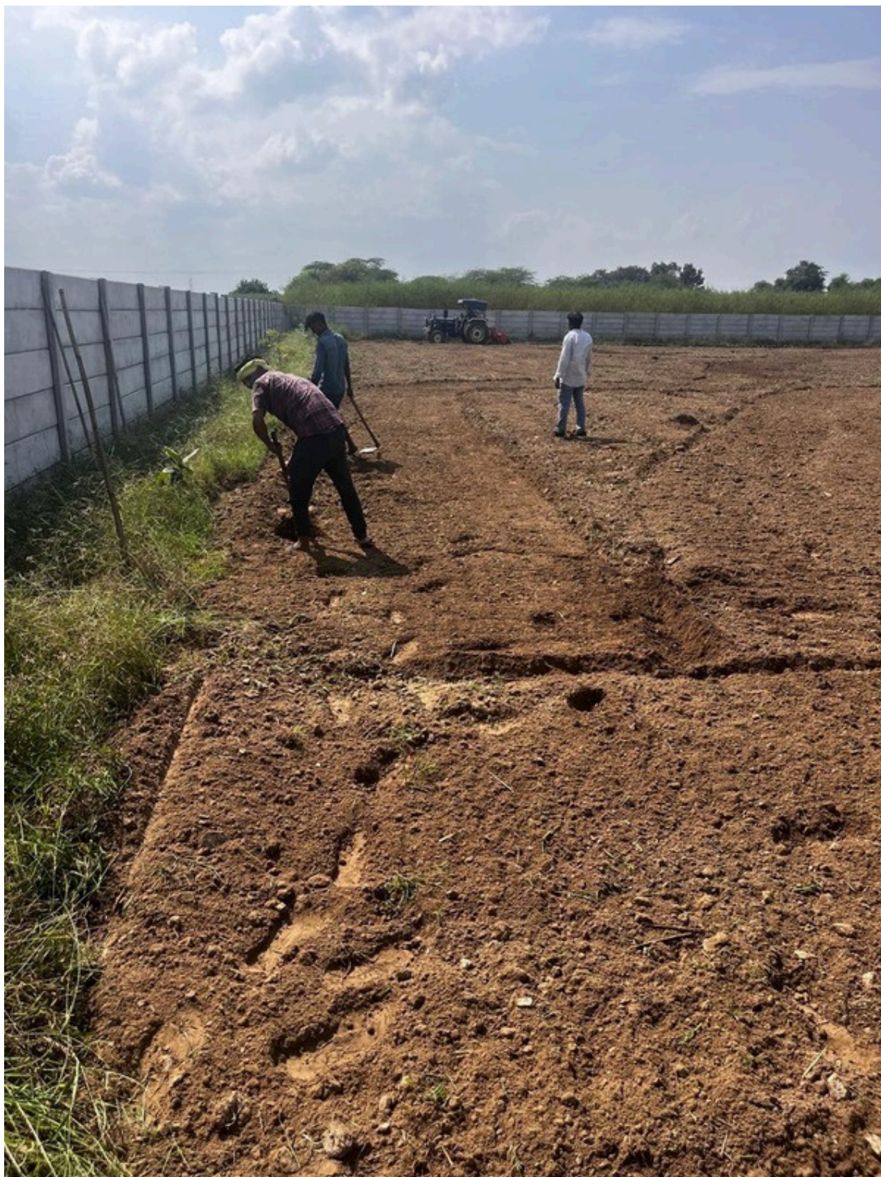
Levelling of Land Post Mixing of Biomass with Soil
