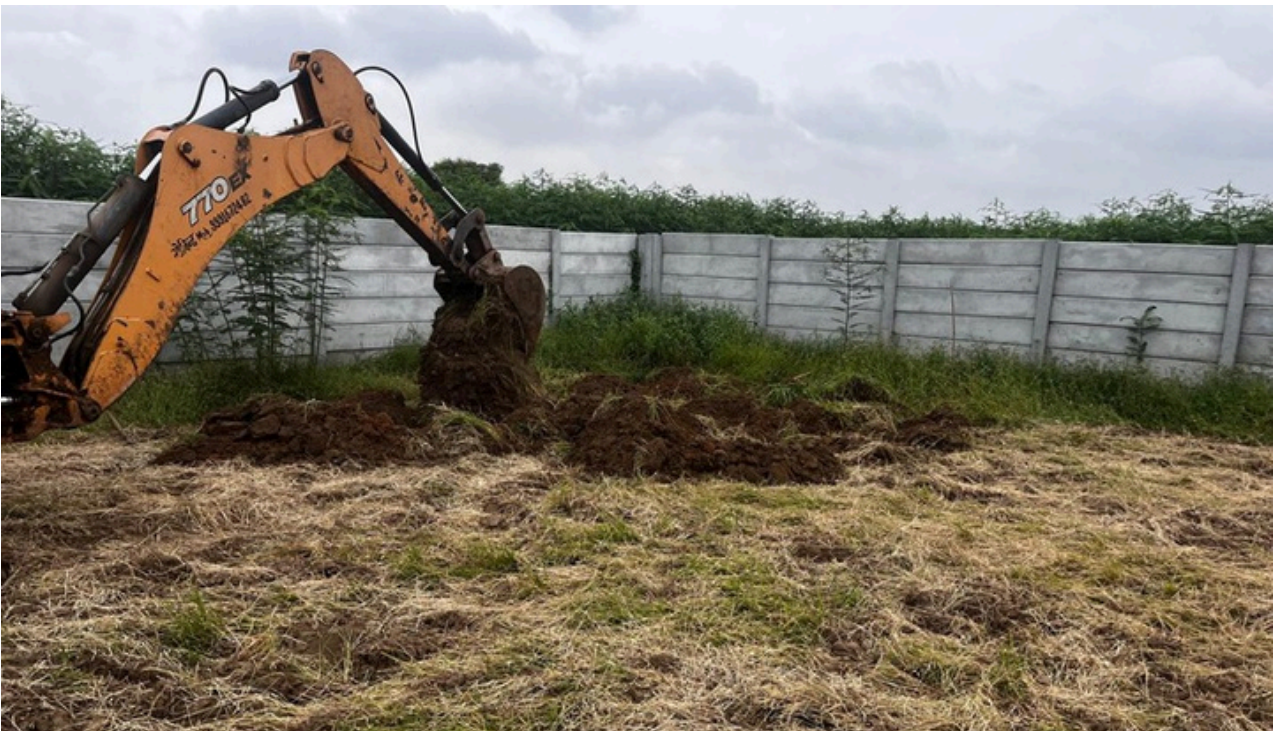
Land Clearing & Levelling
