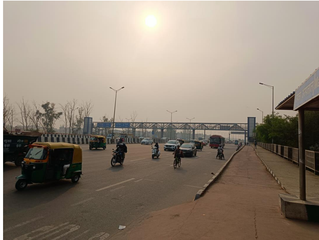
2) Foot Over Bridge Connecting Max Hospital Bus Stop
