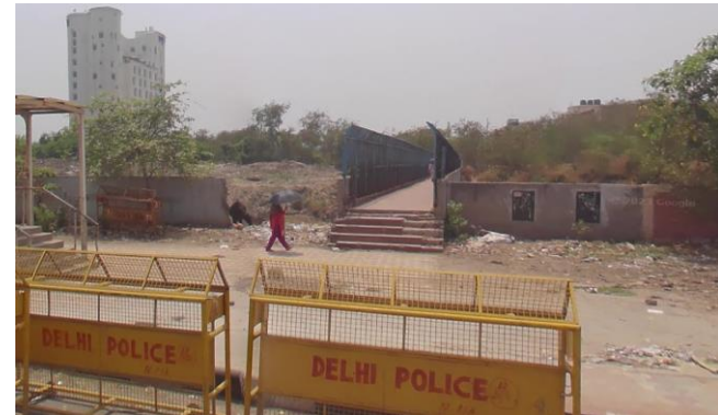
3) Pedestrian Bridge connecting CBSE Office Road
