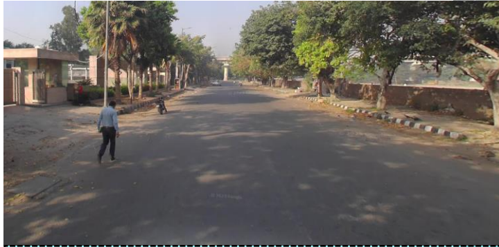
1. Road Marking and signage missing over the stretch having two-way Circulation
