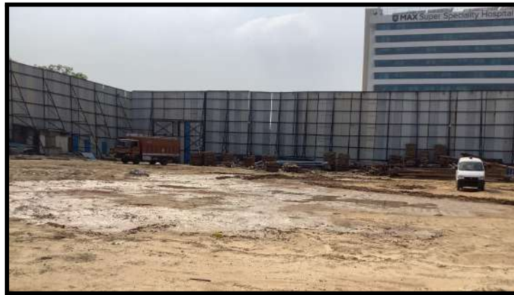
Figure 3. Barricading Around the Periphery of the Project Site
